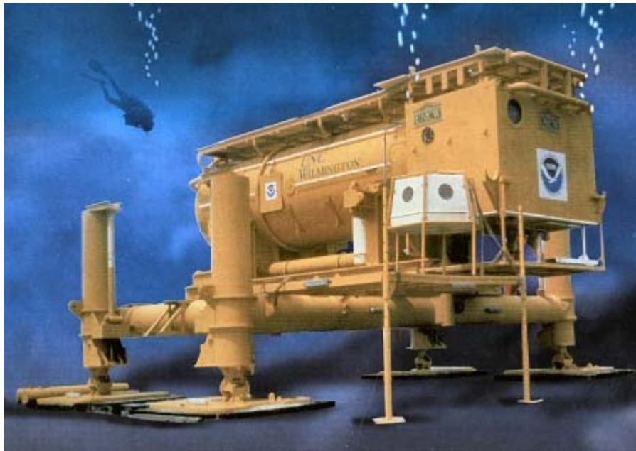
Owned by NOAA and managed by the University of North Carolina at Wilmington (UNCW), the AQUARIUS habitat is an 82-ton double-lock pressure vessel approximately 14 meters long by 4 meters in diameter.
