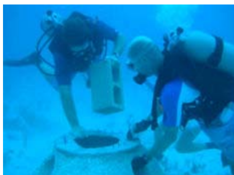
Kilfoyle and Pat Quinn (one of the NSU team) placing cinder blocks into the interior of the artificial reefs to increase internal refuge space complexity.
